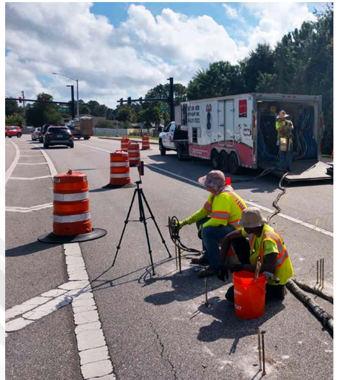
Traffic was diverted, but remained flowing throughout the project
