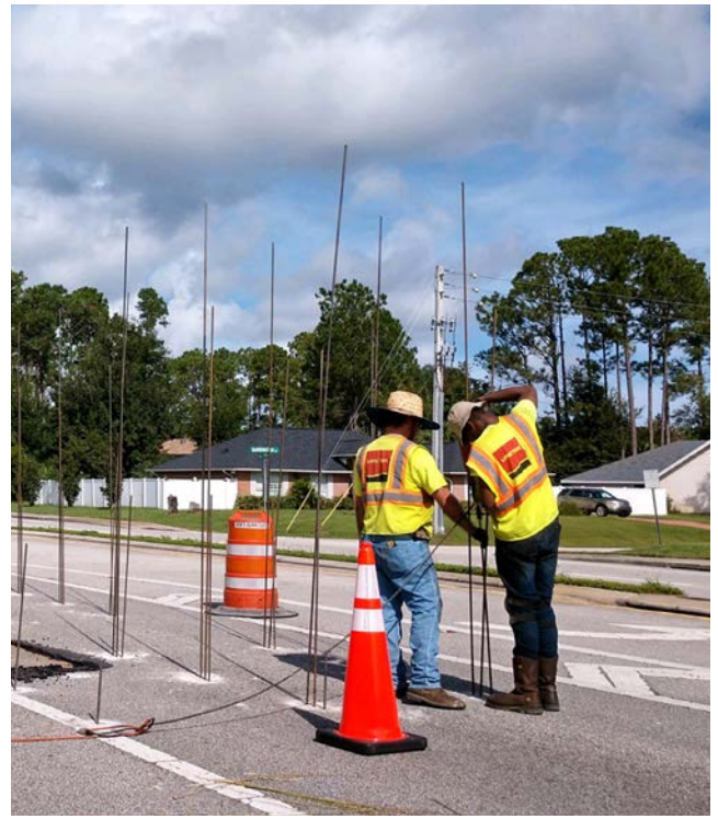
URETEK crew members install injection tubes at the work site
